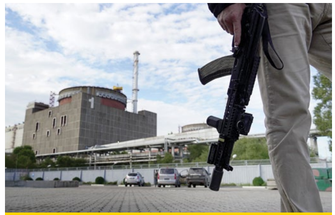
The Zaporizhzhia Nuclear Power Plant, Europe's largest, was captured and occupied by Russian military forces in March 2022. AFP/GETTY IMAGES
