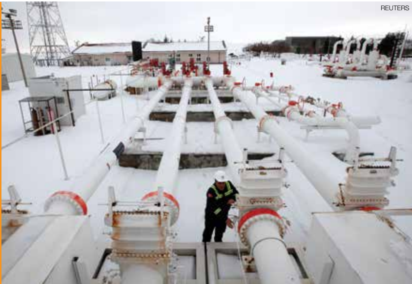
A worker checks valve gears at a natural gas control center at Turkey's Petroleum and Pipeline Corp. Turkey hopes to become a major transit hub for European shipments of Central Asian gas.
